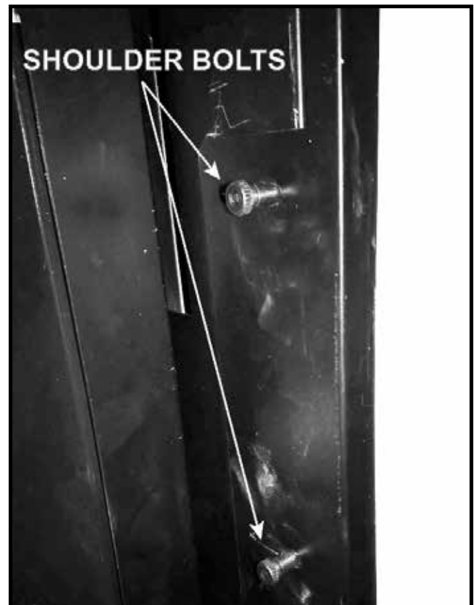
Figure 8. Shoulder Bolts Installed
