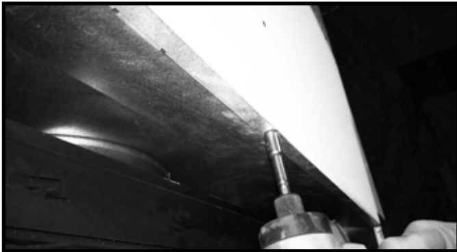
Figure 5. Remove Screw from Top of Appliance Opening
