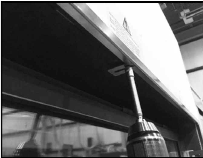
Figure 6. Install Trim Ring
