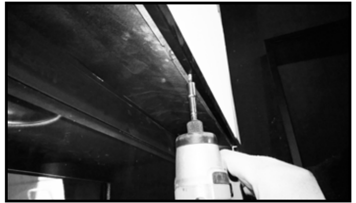
Figure 6 Install Screws in Trim Ring
