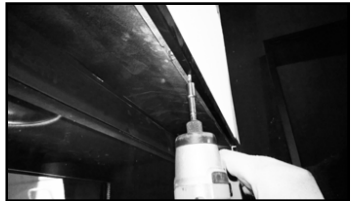
Figure 6 Install Screws in Trim Ring
